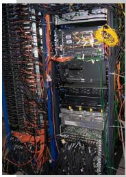
The communications rack: central InfiniBand switches (bottom) connecting nodes and storage servers and the connections to the 20 Gbps CRN (top).
